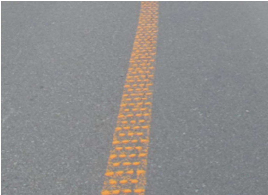
Fig. 13. A high visibility road marking
